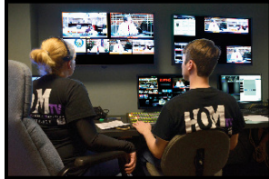
New Master Control Monitors
